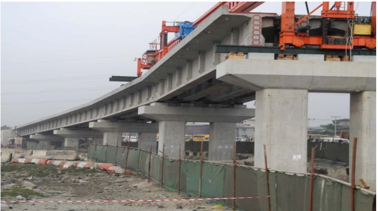
Lagos Light Rail Works Credit: www.nanngroonline.com
