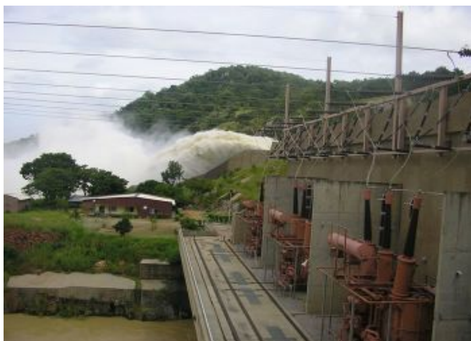
Shiroro Hydroelectric Power Station
